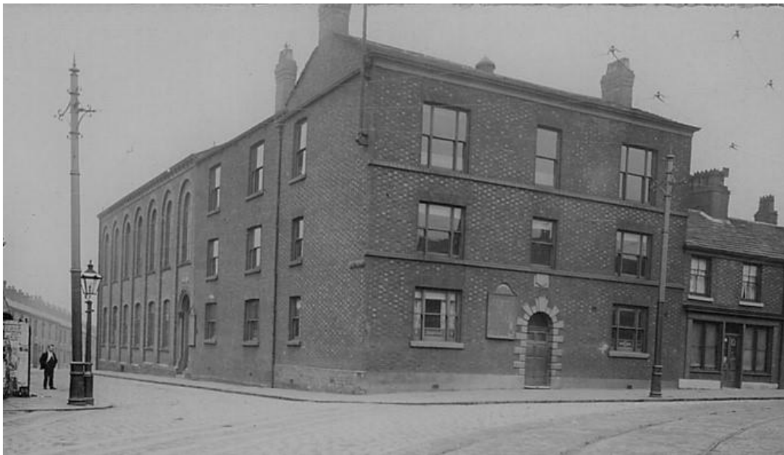
The same view of the school in an early 20 th century photograph
